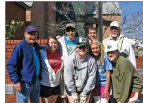
Members of NAILS—the student arm of Laborers For Christ—from Concordia University Texas, Austin, and Slidell, La., joined Laborers and congregation members of Bethany Lutheran Church, Slidell, during their spring break to help construct a new Open Arms Child Development Center.
